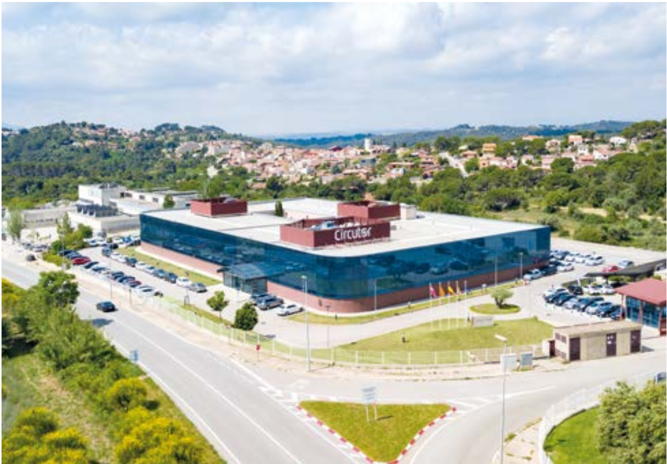
CIRCUITOR headquarters in Viladecavalls, Barcelona.
