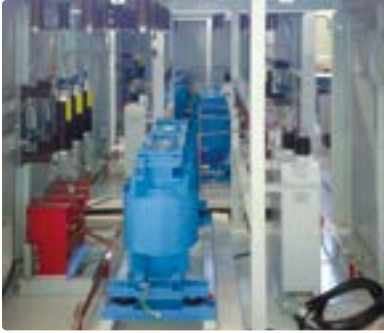
Water treatment installation
